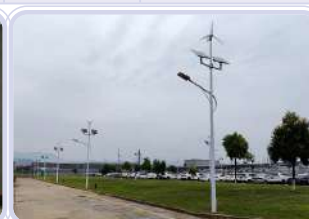
Hybrid wind-solar street lights
